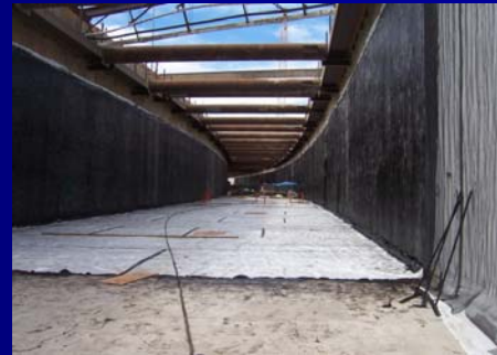
Waterproofing Applied
