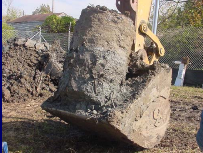
Extraction of Column
