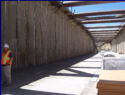
Exposed Soil-Cement
