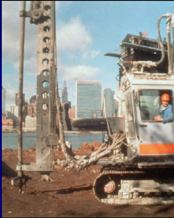
First Dry Mixing Project Queens, NY (1996)
